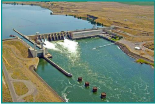
The Ice Harbor Dam on the Snake River is one of four in southeastern Washington that have been at the center of debate for decades.
